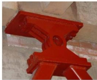
Round hole and Double X-shaped devices (Li et al., 2014)
