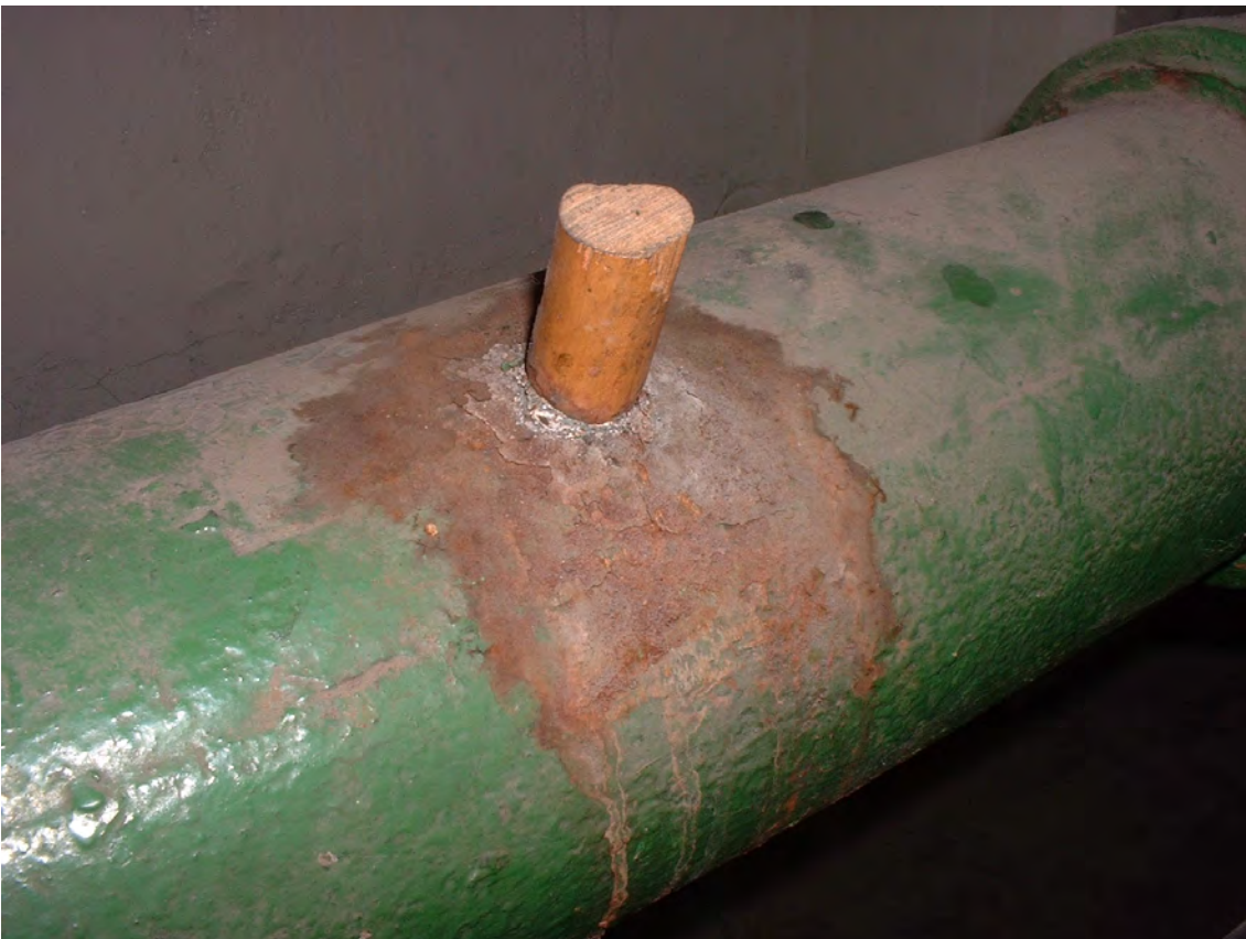
Figure 5: Replacing a small part of a line. Photo credit: Corrvew.
