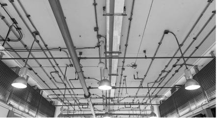
"A fire sprinkler system is an active fire protection method, consisting of a water supply system, providing adequate pressure and flowrate to a water distribution piping system, onto which fire sprinklers are connected."
