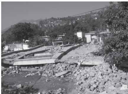
Masonry House, Muzaffarabad
