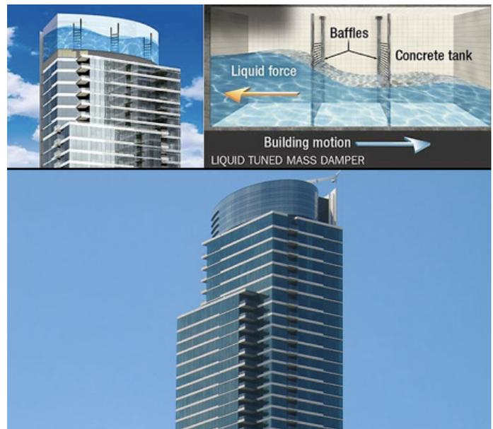
Example of a Liquid Damper installed on a high-rise building (Source: <http://www.techeblog.com/>)
