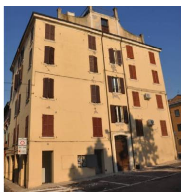
Figure 1. URM façade with a regular opening layout [1]
