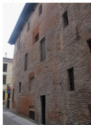
Figure 2. URM façade with an irregular opening layout [1]
