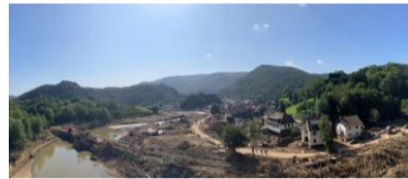
Figure 2. Flood damage in the Ahr valley, July 2021 (photo by Dr. Holger Maiwald)
