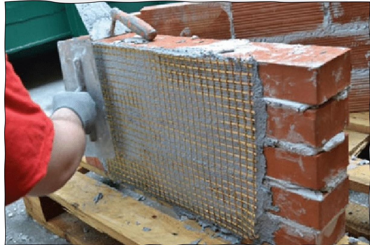
Figure: FRCM application to masonry wall
