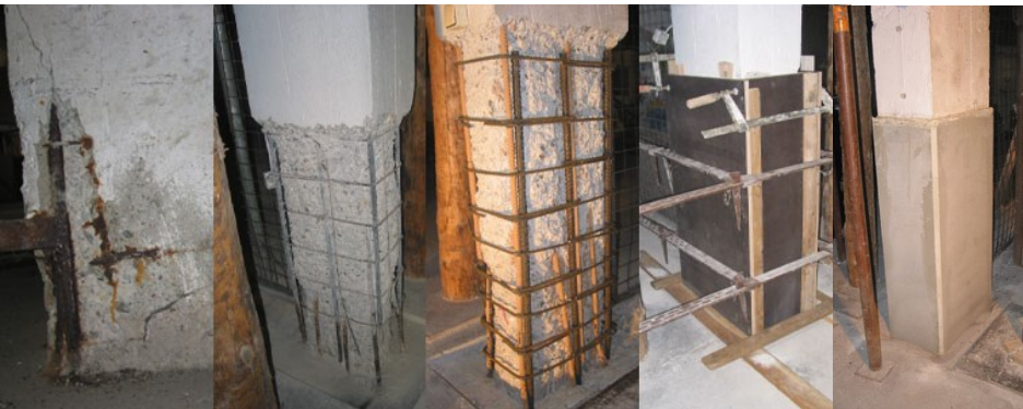
Fig. 1# Example for application PCC
