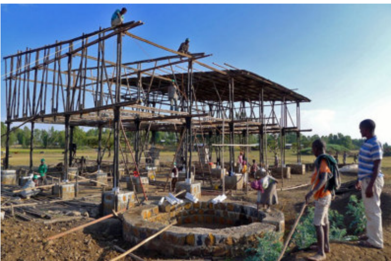
fig. 2.15: community construction work in Buranest, part of NESTown project. (Hefti 2012)
