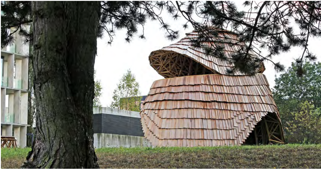
Figure 2.10: Exterior image showing the shingle pattern and opening sequence of the structure. Photograph by Philipp Eversmann et al., 2017.
