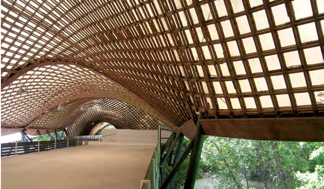
Figure 2.8: Multihalle Mannheim, Gridshell . Photograph by Eberhard Möller, 2015.
