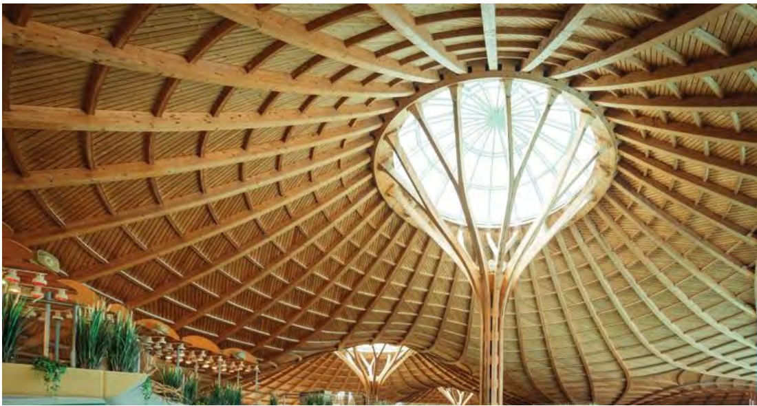
Figure 2.14: Tree columns at the Bad Dürrhein brine baths . Photograph by Kur- und Bäder GmbH Bad Dürrhein, 2016.
