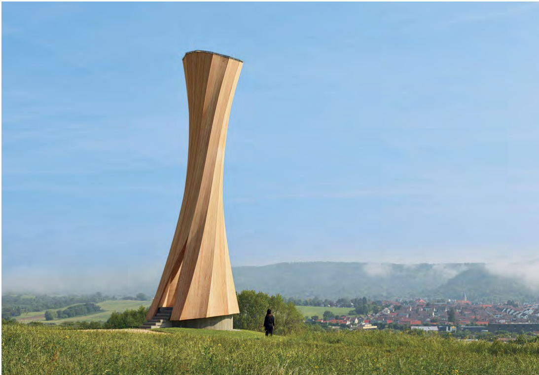
Figure 2.12: The Urbach Tower, a high performance timber structure utilising self-shaping wood manufacturing for curved CLT. Photograph by Rolland Halbe, 2020.
