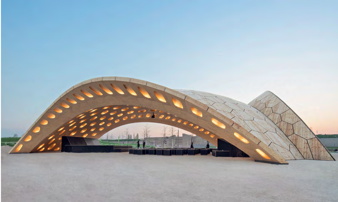
Figure 2.9: View of the BUGA Wood pavilion with illuminated hollow chambers of the structural cassette segments. Photograph by ICD/ITKE University of Stuttgart, 2020.
