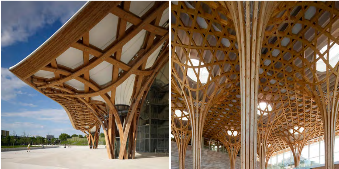
Figure 2.15: Left: Centre Pompidou-Metz . Right: Haesley Nine Bridges Golf Club House . Photographs by Shigeru Ban Architects, 2010.
