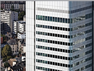
Silvertower, Frankfurt am Main schneider + schumacher
