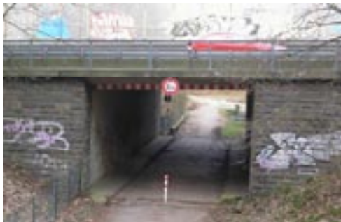
Figure 6. Reinforced concrete slab bridge
