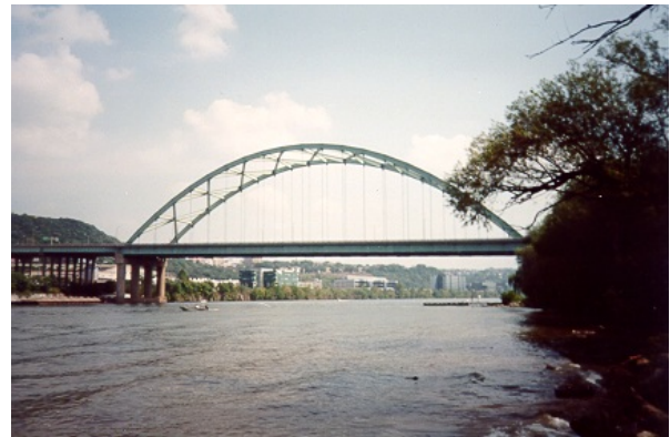
Figure 5.47: Birmingham Bridge, Pittsburgh, Pennsylvania, USA.
