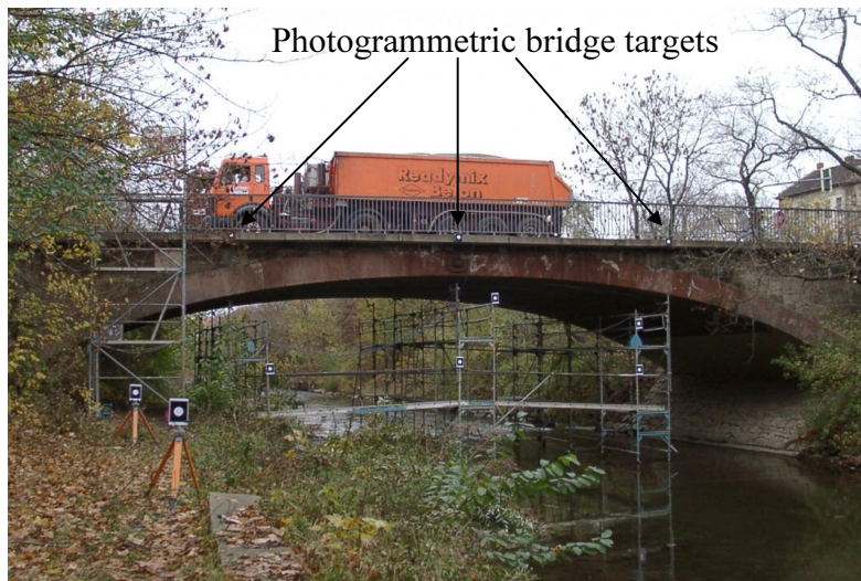
Figure 8: Franckebrücke at Erfurt with the trestle for fixing the inductive gauging sensors, the targets for the photogrammetric measurement and the trucks
